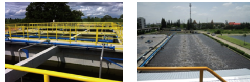
AC industry complex and AN industry complex in Thailand
