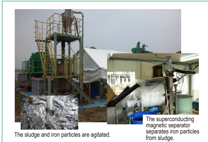
Separation/removal of arsenic from the sludge using functional iron particles.
