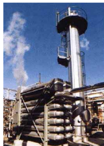
Appearance of system for ethylene plant
