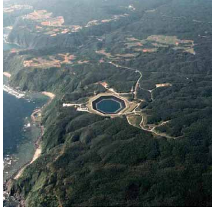
Okinawa seawater pumped-storage power plant
