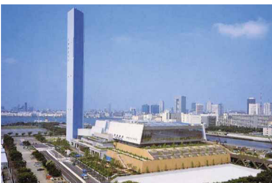
Chuo incineration Plant (Chuo-ku, Tokyo)
