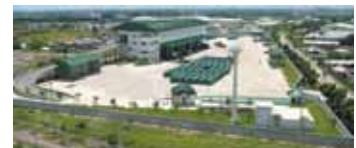
Waste Transfer Station at Nongkhaem, Bangkok
