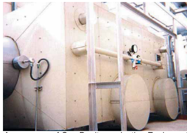
Appearance of Gas Denitrogenization Equipment (SCR Reactor)
