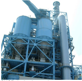
SNCR denitration equipment (Urea solution system)
