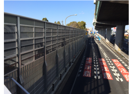
An example of NNC panel installation
