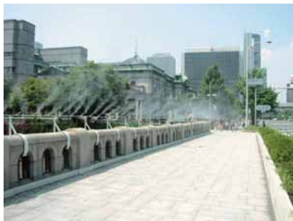
Dry misting using water that has been treated by advanced purification (Yodoyabashi Bridge)
