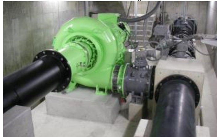
Small-scale hydropower generation system (hydroelectric generator), Sakurai Water Treatment Plant
