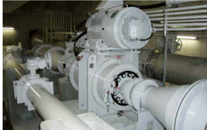
Small-scale hydropower generation system (hydroelectric generator), Nara Prefecture Regional Waterworks Center
