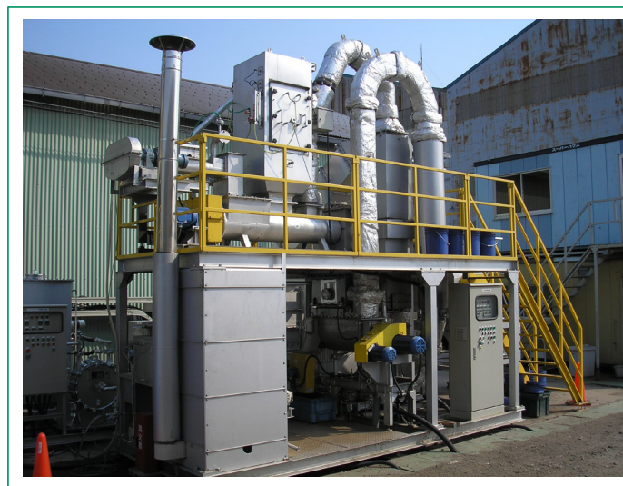
External view of the system
