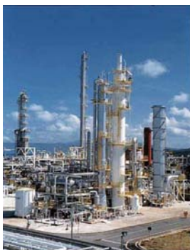
CO 2 recovery plant
